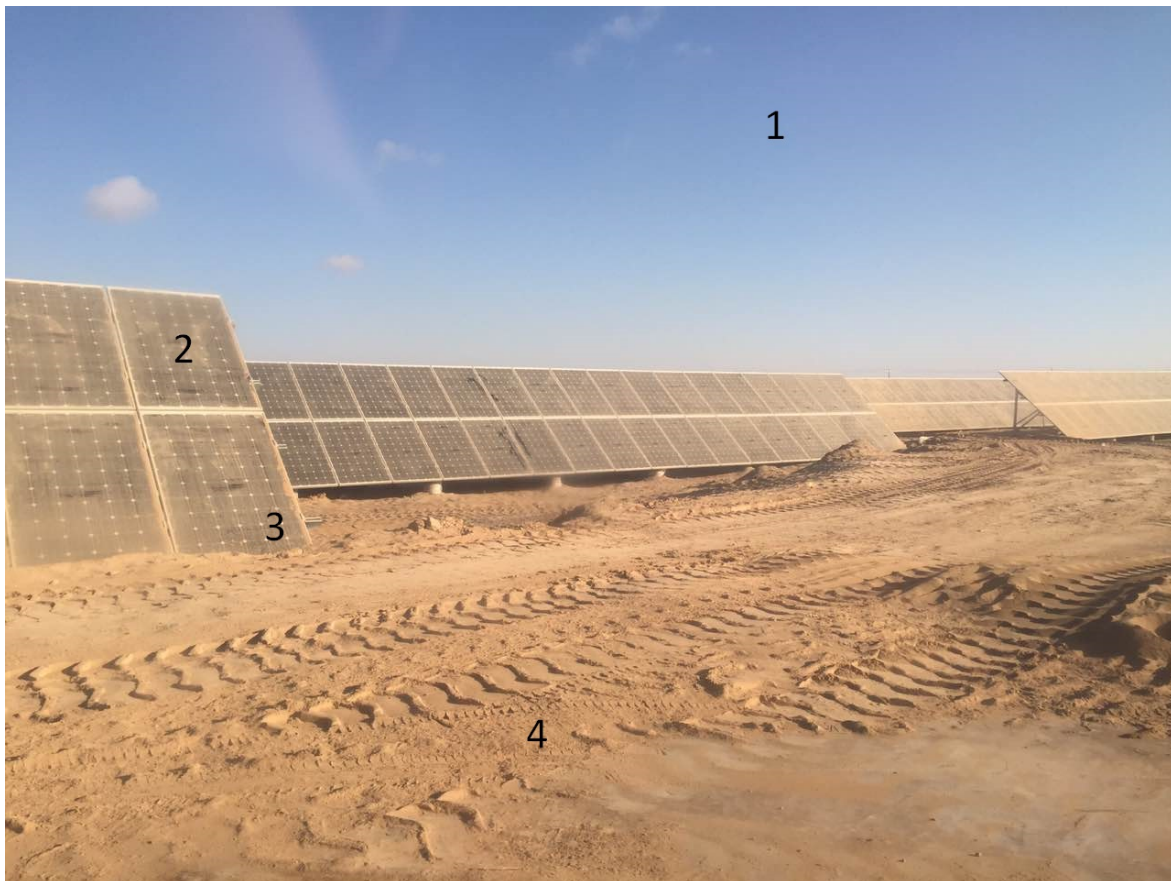
Fig. 32: Factors influencing dust soiling of PV modules in desert regions: 1 Climatic impact, ambient dust concentration, 2 Glazing characteristics, adhesion effects, non-uniform soiling, 3-Installation conditions, 4-Surrounding environment, dust particle characteristics. Photo: TÜV Rheinland Group
