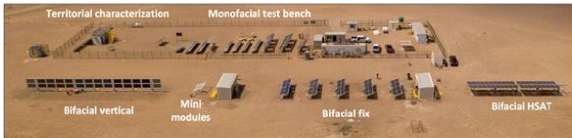
Figure 39: Current facilities at the Atacama Desert solar platform.
